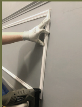
❸ You can also nail the frame line to the wall with a nail gun
