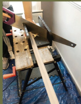
❶ Cutting Moulding With cutting machine
